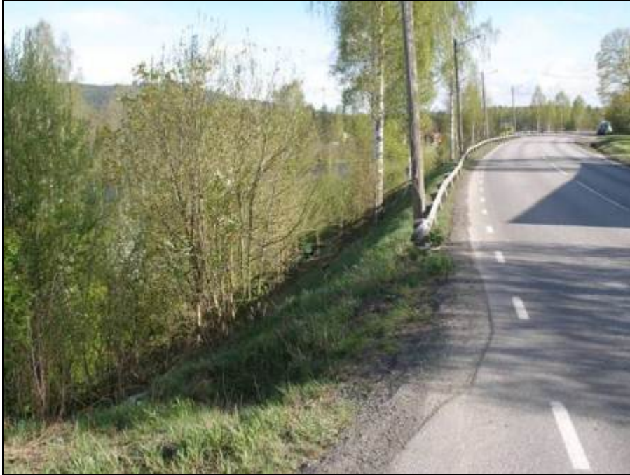
Figure 20 Approach Photo Example
