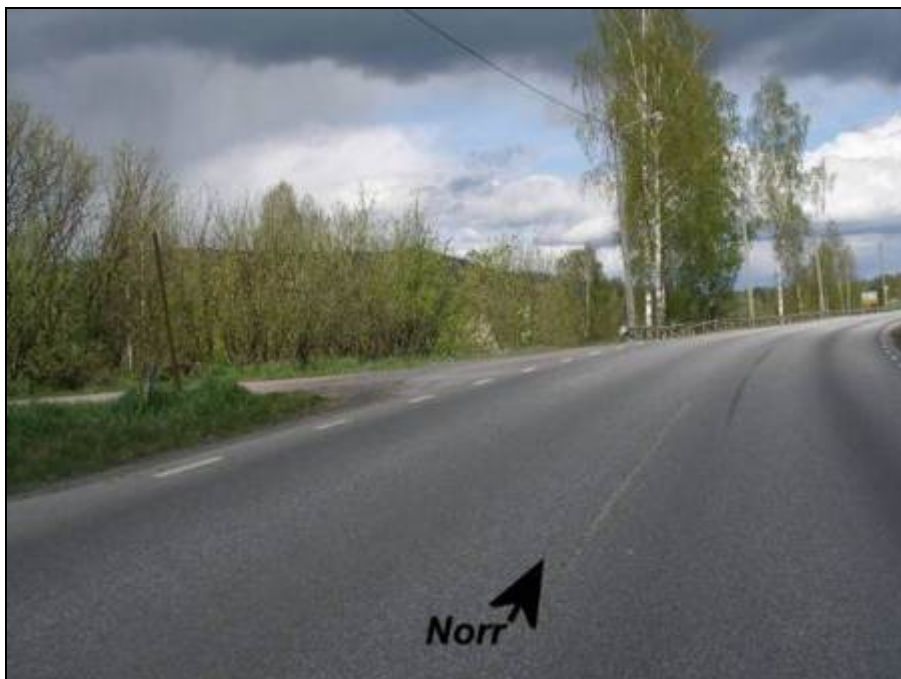
Figure 19 Approach Photo Example
