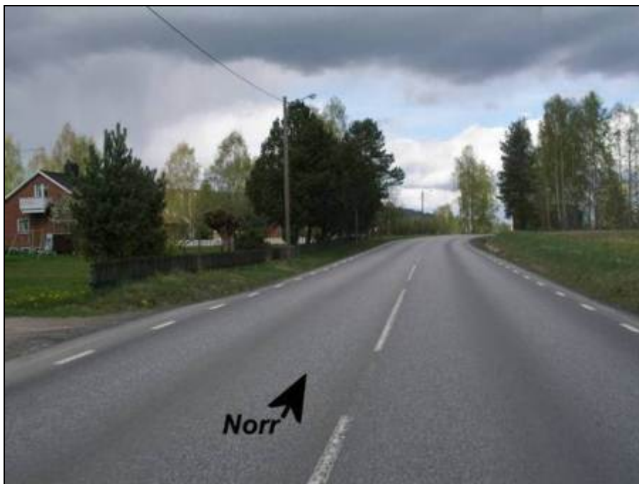
Figure 17 Approach Photo Example
